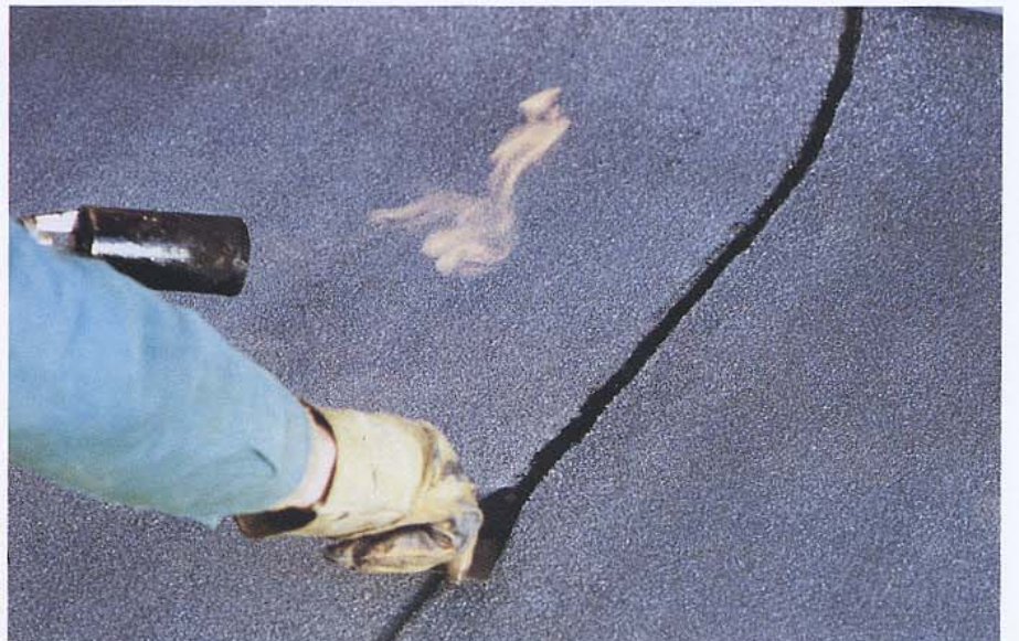
Sealing the overlaps using a rounded trowel.
